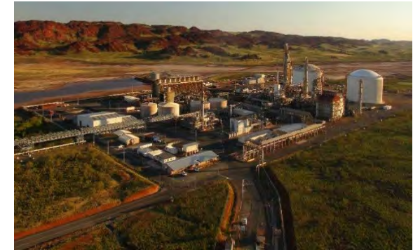
Green Molecules Turnkey Integration, Electrolyzers, Project Development & Asset Management
